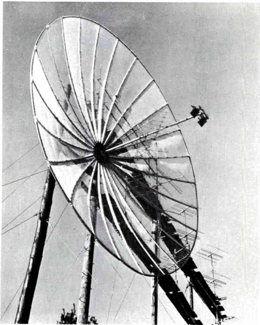
RF Systems' parabolic antenna for CATV reception
