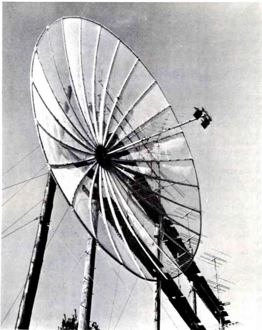
RF Systems' parabolic antenna for CATV reception
