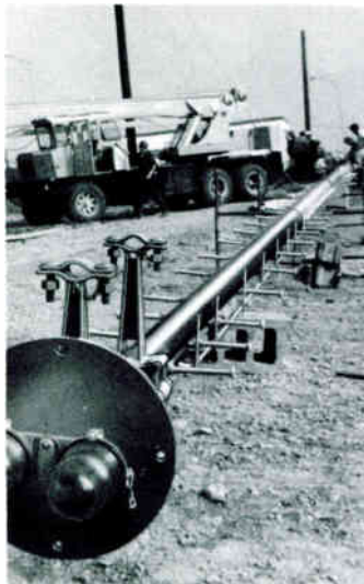
Pole and accessories assembled on ground prior to erection.
