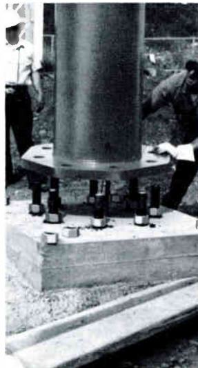
Pole in position to be lowered on plumbing nuts.
