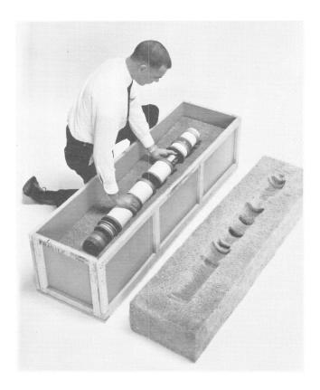
Figure 10—Storage of Klystron in Shipping Crate.
