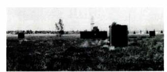
Figure 2 Chain link fence with redwood slats was used around the tower base and at each of the three guy anchors.
