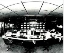
NBC's Skypath facilities include a Satellite Network Management System for control of 356 antennas, 794 receivers, and 378 computers at the earth stations of 175 NBC-TV affiliated stations.
