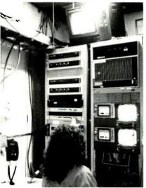
M/A-Com satellite receivers mounted adjacent to waveform monitors in the transmitter control area at KOB-TV, in Albuquerque, NM.
