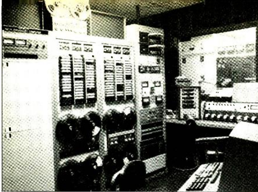
Main control room, automation in center, console to the right. Cart player is to left of console
