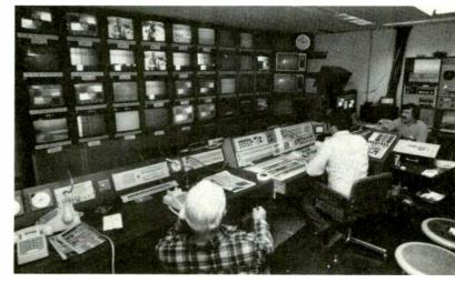
Production control room B at proadcast center with Grass Valley 1600 7K switcher and Vital four-channel SqueeZoom. Audio position, identical to control room A, had Ampex reel-to-reel and ITC cart decks
