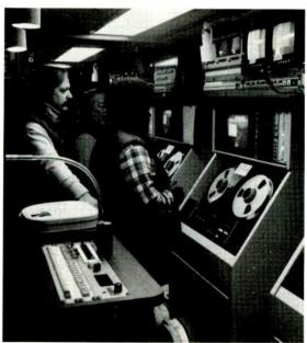
Matched half of Phase 8 videotape van with Ampex VPR-2s. In separate compartment are HS slow mos, and, in another compartment, Chyron character generators
