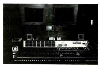
At the front of interior is the Ward-Beck console, which provides mixdown from up to 32 microphone inputs, or from the 16 tracks of Ampex recorder
