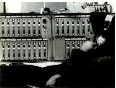
Production coordination intercom system located in control room A. Operator-assisted, it linked 57 remote locations with six trunks handling up to 10 conversations per trunk
