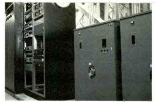
Transmitters are in seventy-fourth floor penthouse of central hotel tower, just under the roof. The antenna is directly above, so transmission line can come straight down
