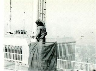
Rigger completes work on Bogner four-bay slot-and-dipole CP antenna for WTVG's 1000 W translator in south tower of World Trade Center, 1,398 feet above sea level. Note in background the north tower mast which will house an array of VHF antennas for the New York area
