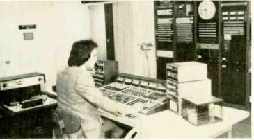
Master control for new Mutual system includes switching for routing incoming material to one of taping rooms or "on air," plus switching for outgoing feeds, ordinarily assigned by the computer. Console also has keyboard for entry of additional program events in computer memory; with have CRT read-cut of program block (not installed at time of picture).
