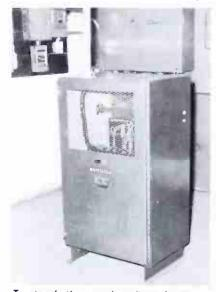
To steady the supply voltage for a mountain-top transmitter at the end of the power line, WBRE-FM installed this self-contained Solartron regulator; it keeps the output power within FCC limits. mitter site. When operations cease for the lunch hour at the close of the day, power surges. An hour later we area residents start preparing the evening meal switching on TV and lights, the power drops again. It later on there's another increase as Wilkes-Barre refor the night.
