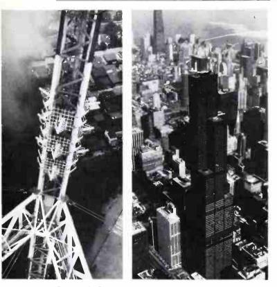
Fig. 8, left. FM version of the CP antenna, long used, is shown in photo on leg of Mt. Sutro Tower in San Francisco, where it serves for high-power transmission. Fig. 9, right. CP antenna got on-air tests at Chicago station WLS-TV, mounted atop the worlds-tallest Sears Building as shown here.
