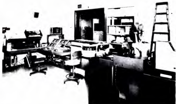
Cable control room, next to two-story studio, has switching in front of studio window. Norelco LDH-1 film chain at the right. IVC 1-inch and Sony 3/4-inch cart machines are primary sources of recorded video programming.
