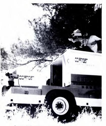
Camera-studio truck operating with camera on roof, another on open rear platform. Complete control studio is inside roofed part of truck. Power truck can be seen in background. bank, California. Aiming for very compact, easily operated units that get into action quickly, Compac built the studio into a van-type vehicle with a overall length of 20 ft 2 in., and the power suppl into another truck only 16 ft overall.
