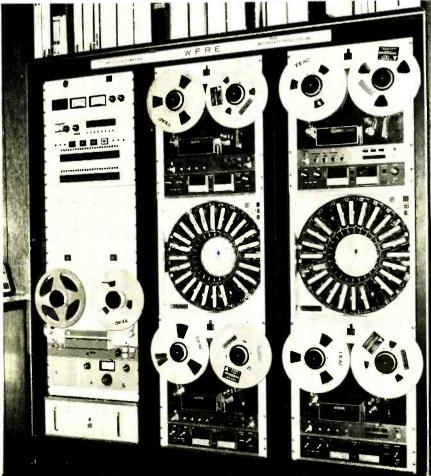
Automation at WFRE. Rack at left includes, from the top, silent sense unit, VU monitoring panel, digital master clock and timeactivated control circuit. slow-speed audio logger, and, at the extreme bottom the automatic time announcer. The automatic network delay cart to extreme left was cropped out of photo. Four reelto-reel music transports and two carrousels make up the two remaining racks.
