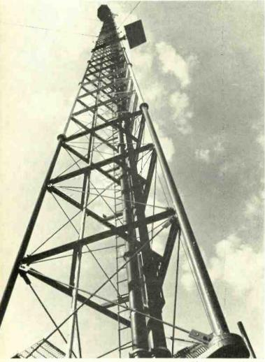
To increase power output from 60 kW to 120 kW, Channel 61, Cleveland, is replacing the  $6 \cdot \frac{1}{8}$ -in. coaxial transmission line shown here with a new  $6 \cdot \frac{1}{8}$ -in. line using "Freon" HFE coaxial cable gas. The HFE line means an increase in power output with no additional increase in size or weight and no effect on wind loading of the tower.
