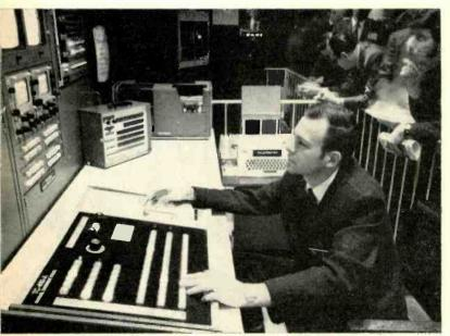
You can use a mini-computer to do most in-station jobs such as controlling video switching. The GE/PAC-30 can take over this man's job.
