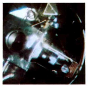
Early in this flight, this transmission showed the Lunar Module, still attached to the Saturn IVB stage. This picture was transmitted before the LM extraction from the booster rocket. Circular object is the docking drogue assembly.
