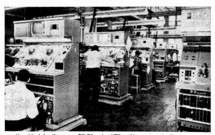
Yes, Virginia, there are TR-70 color VTRs. Shown here in final test are TR-70's shipped last December. The \$82,500 "high band" machines undergo 240 hours of testing prior to release. The TR-70 was introduced at last year's NAB show.
