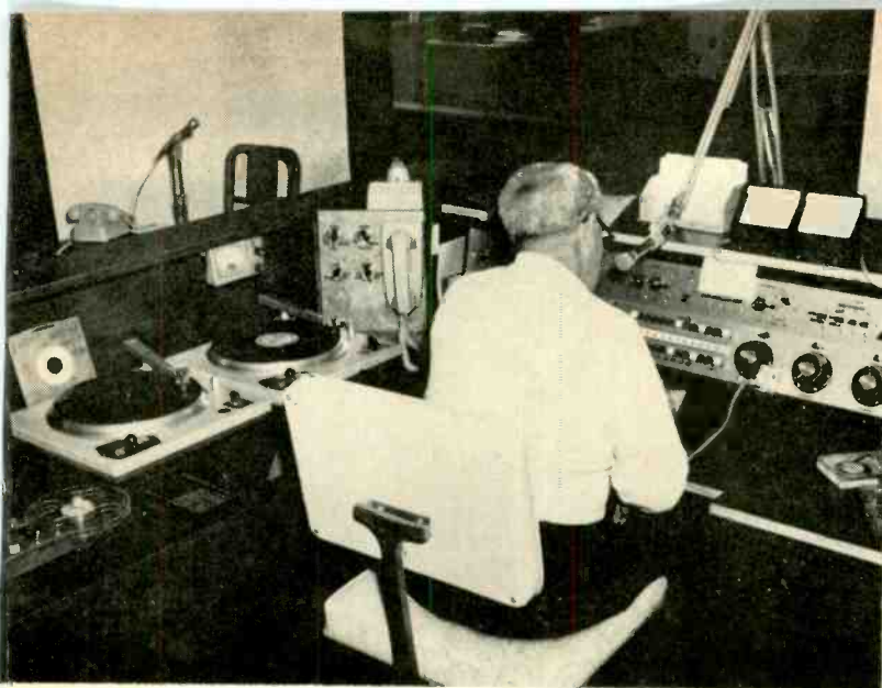
Chief Engineer George Kelly at the master control console. Monitor panel switches on left select network, mobile receiver, or program lines 1 and 2.
