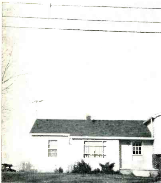
Typical house drop. Lafayette Cable offered to take down antennas no-charge.
