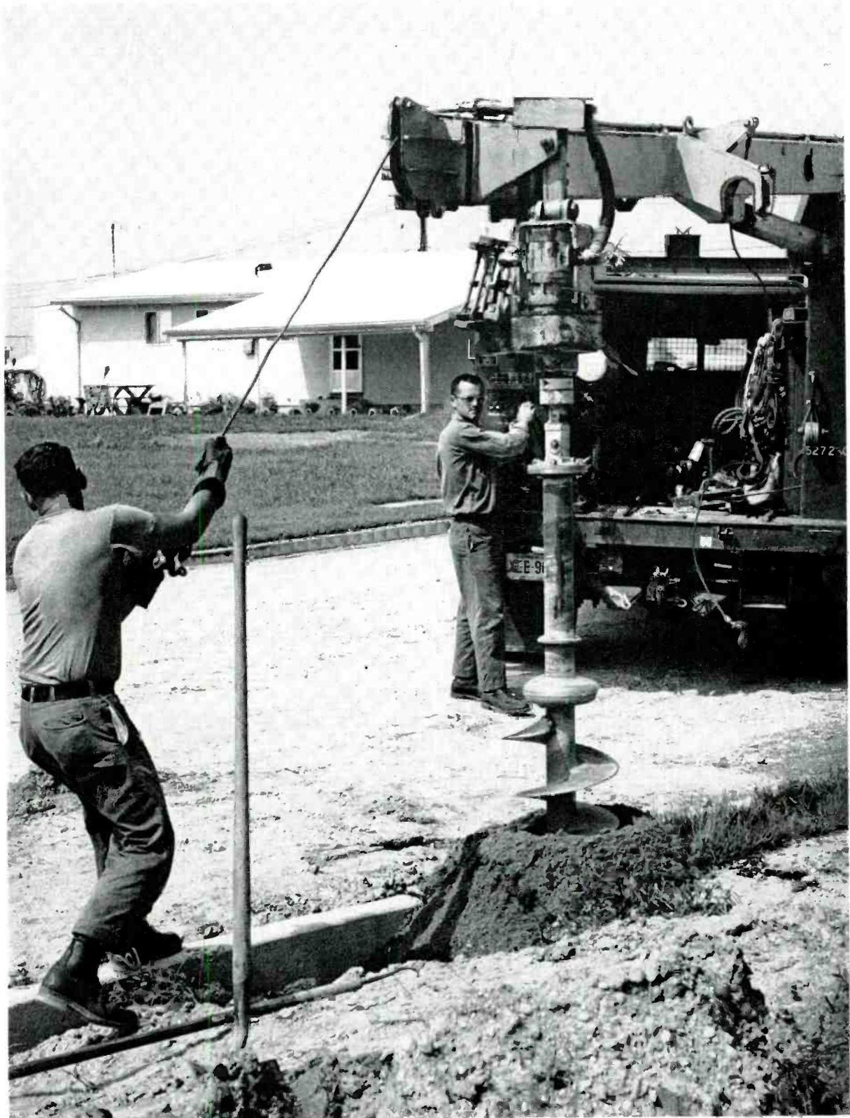
*Two-man crew using construction truck with corner derrick and earth auger to dig telephone pole hole.*
