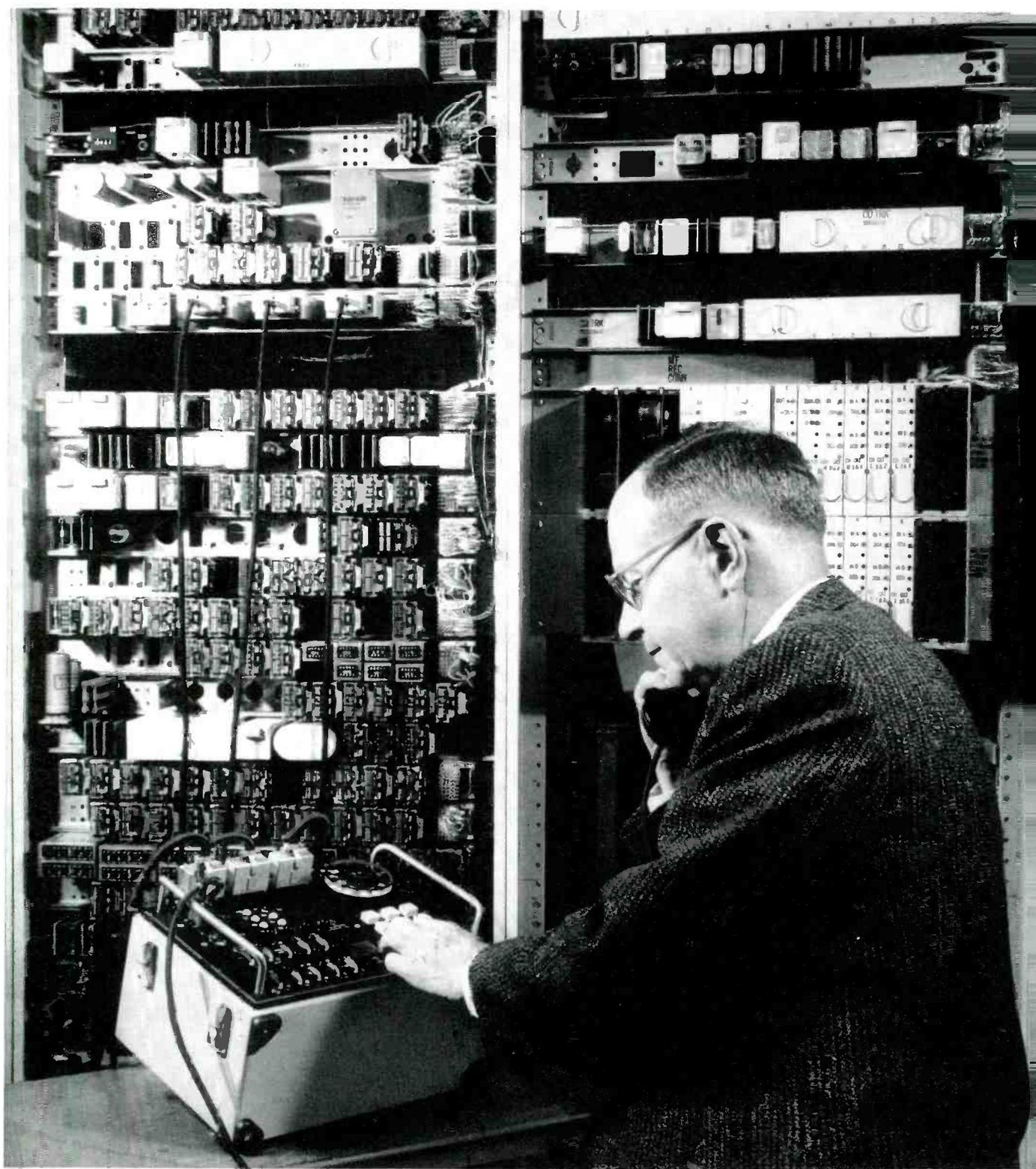
*C. Throckmorton checks operation of the converter circuit for step-by-step with a manual test box. Maintenance testing is accomplished in this manner.*
