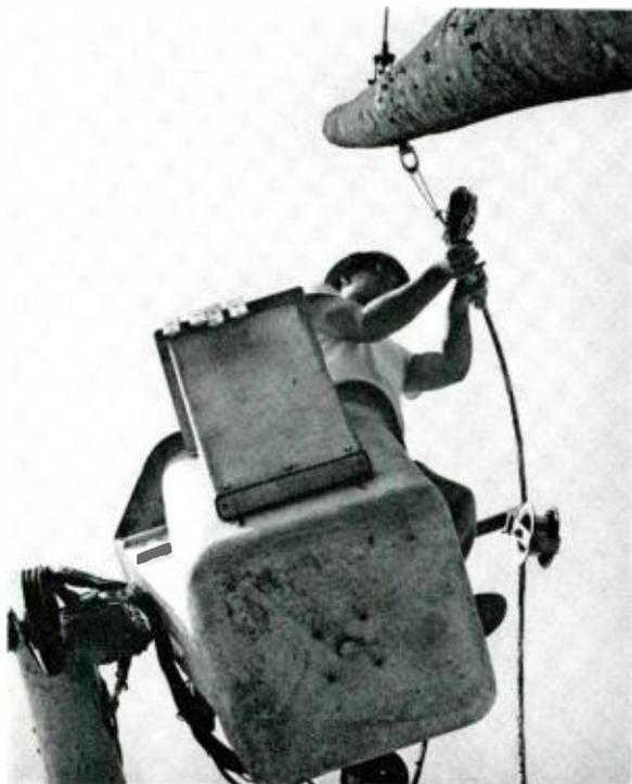
*New Jersey Bell Telephone workman at Neptune, N. J., uses aerial lift to place multiple line wire.*
