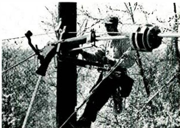
*Fig. 2—The tow truck is stopped when the rear support arm nears the strand support.*
