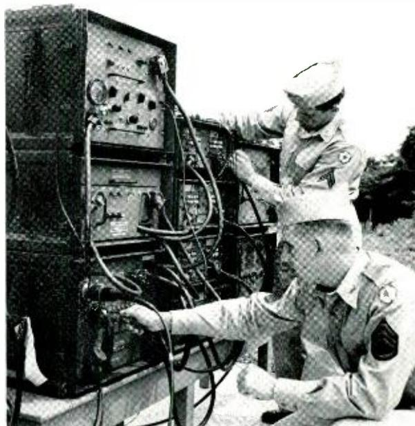
*Army Signal Corps servicemen assemble the terminal units of a new portable twelve-channel telephone system designed for field service by Bell Telephone Laboratories.*
