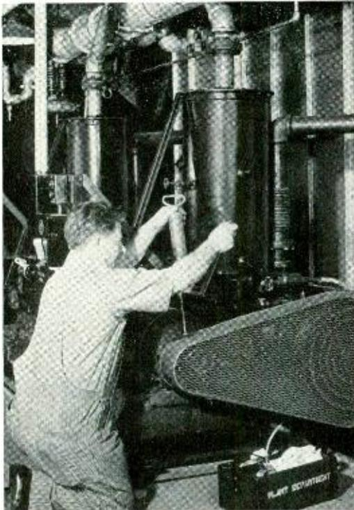
*Fig. 4—These two mechanical vacuum pumps produce the main vacuum in the bell jar and, together with oil diffusion pumps in the base of the plating apparatus, create a vacuum of about 1/10,000 mm of mercury. Mechanic Ralph Coviello is operating the apparatus*
