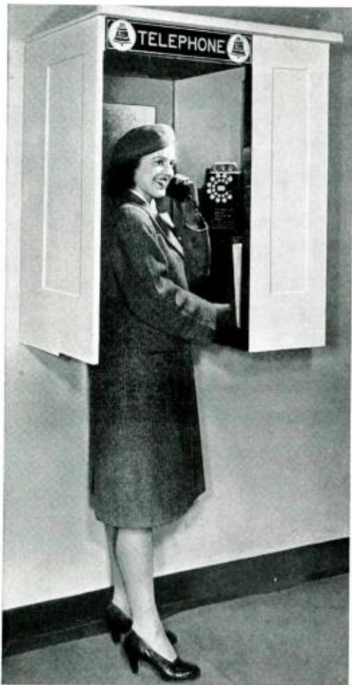
*Another example of wartime streamlining is the semi-booth for public telephones. Designed to be attached to a wall, the new model is expected to be useful in semi-exposed locations, especially in mild climates*
