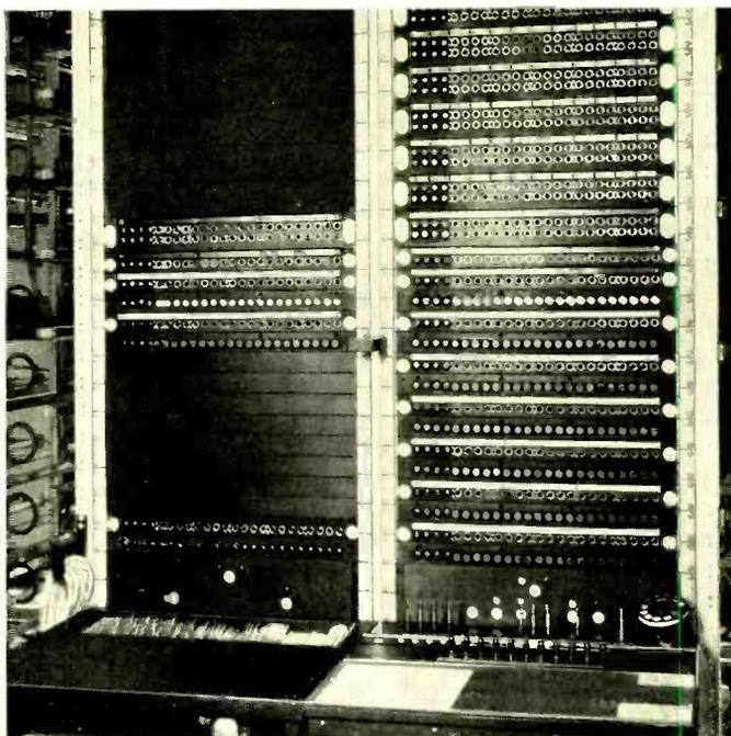
Fig. 5—A non-multiple test and control board at Aurora, Illinois, typical of equipment for the smaller office. Toll lines are made busy by operating the keys seen below the jacks in the lower part of the right-hand panel
