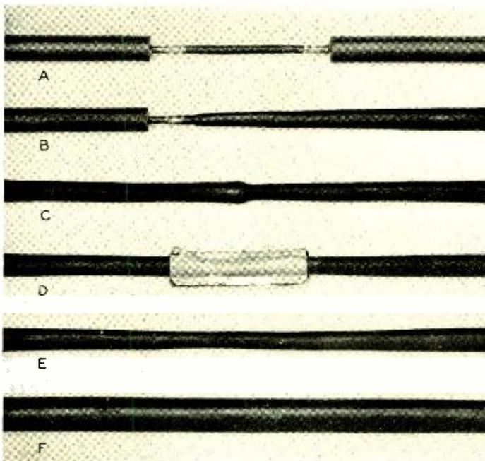
Fig. 4—Steps in splicing paragutta insulation with the aid of the machine
