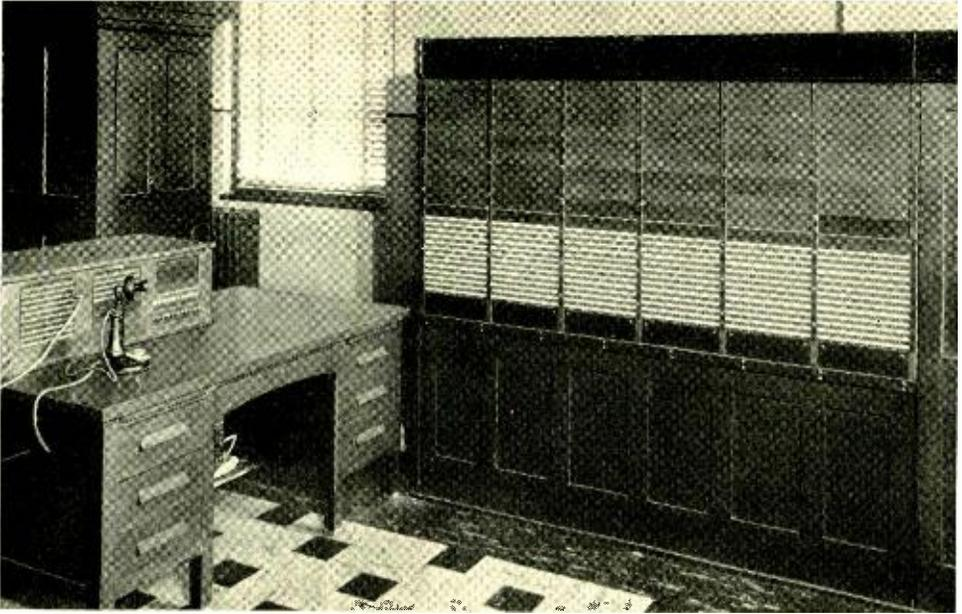
*Fig. 3—Circuit display board which keeps the Traffic Department advised of circuit conditions*
