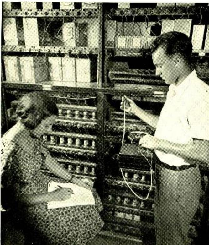
*Fig. 1—Recording voltages of batteries on test in the battery testing laboratory*
