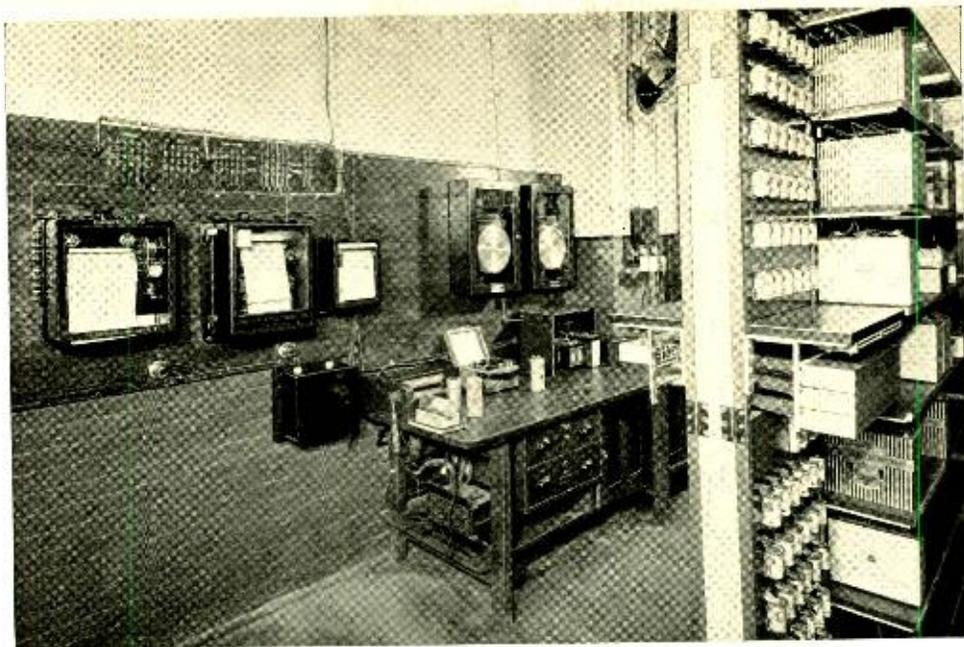
*Fig. 4—One group of program machines and recording meters used for dry cell testing*
