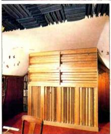
Fig. 6—The dead end of a Live End/ Dead End (LEDE) room in Pisha's home. Front speakers are B & W 801Fs and Janis W1 subwoofers.
