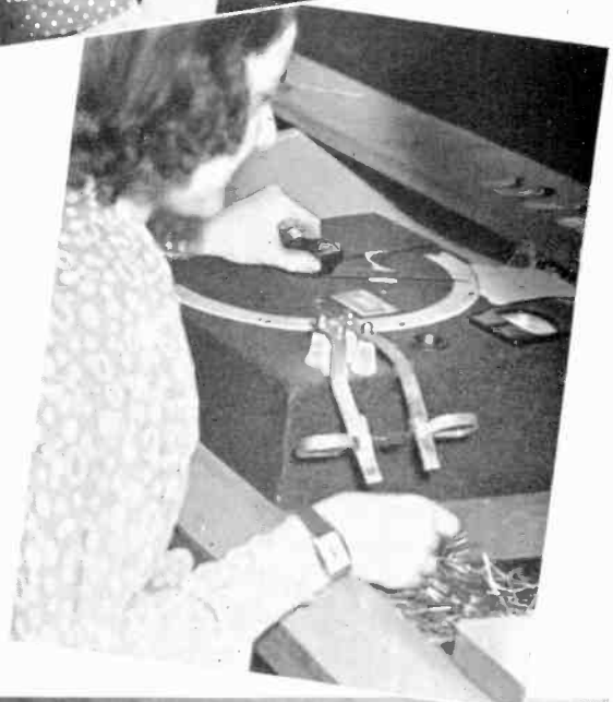
Right: Final test of mica capacitors for capacity and Q.
