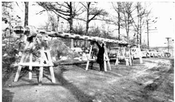
Fig. 11—The RCA TFU-20A UHF antenna in test position before erection on tower.
