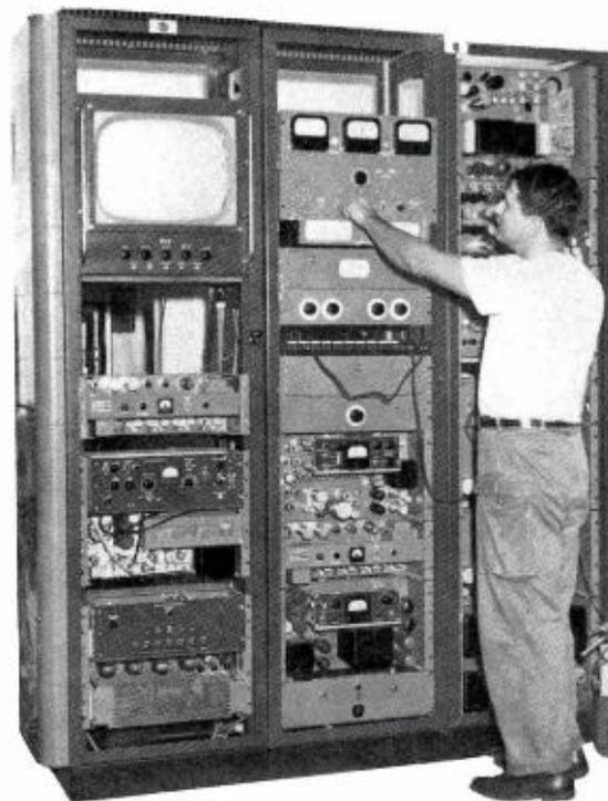
FIG. 18. Microwave equipment in station transmitter room. Left rack: microwave from Roanoke (NBC). Center rack: microwave from Bluefield (STL). Right rack: power supplies.
