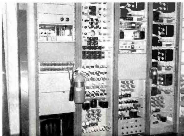
FIG. 4. Equipment racks in studio control room.
