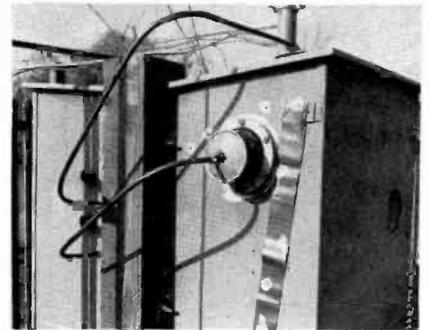
FIG. 14. Tuning houses back-to-back for day-to-night pattern tower.
