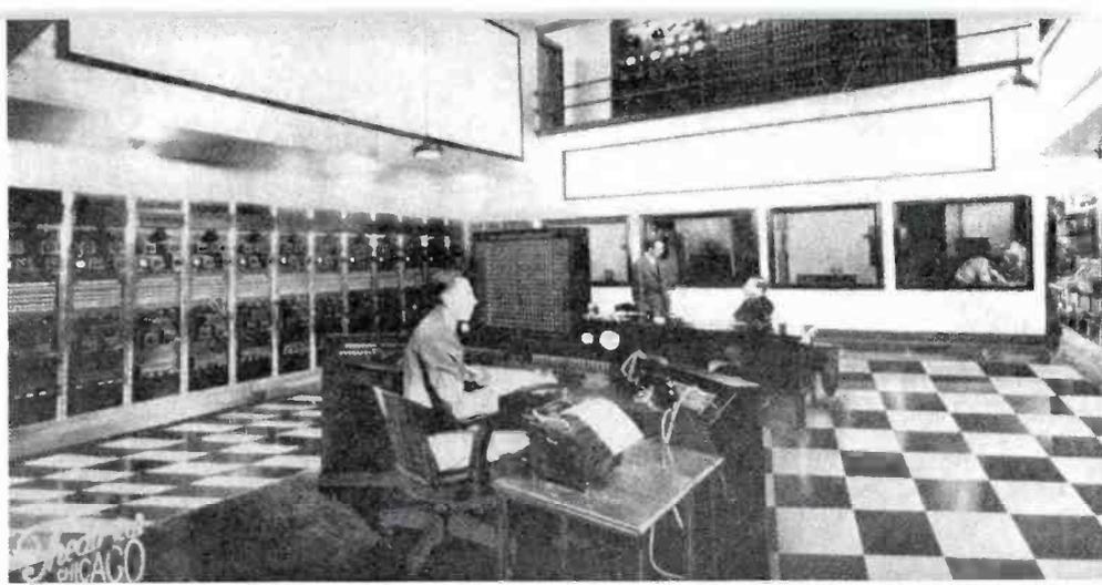
FIG. 3 (top). This picture (reproduced from an illustration in *BROADCAST NEWS* No. 3, April 1932) shows how the old Radio-Master Control of the Chicago NBC Studios looked in the days when it was the awe-inspiring wonder of the just-dawning electronic age. Nostalgic old-timers will recognize (but not weep for) the rows and rows of battery-operated "speech input" equipment. Battery-charging equipment alone required a control panel (balcony) larger than that of a 50 KW transmitter.
