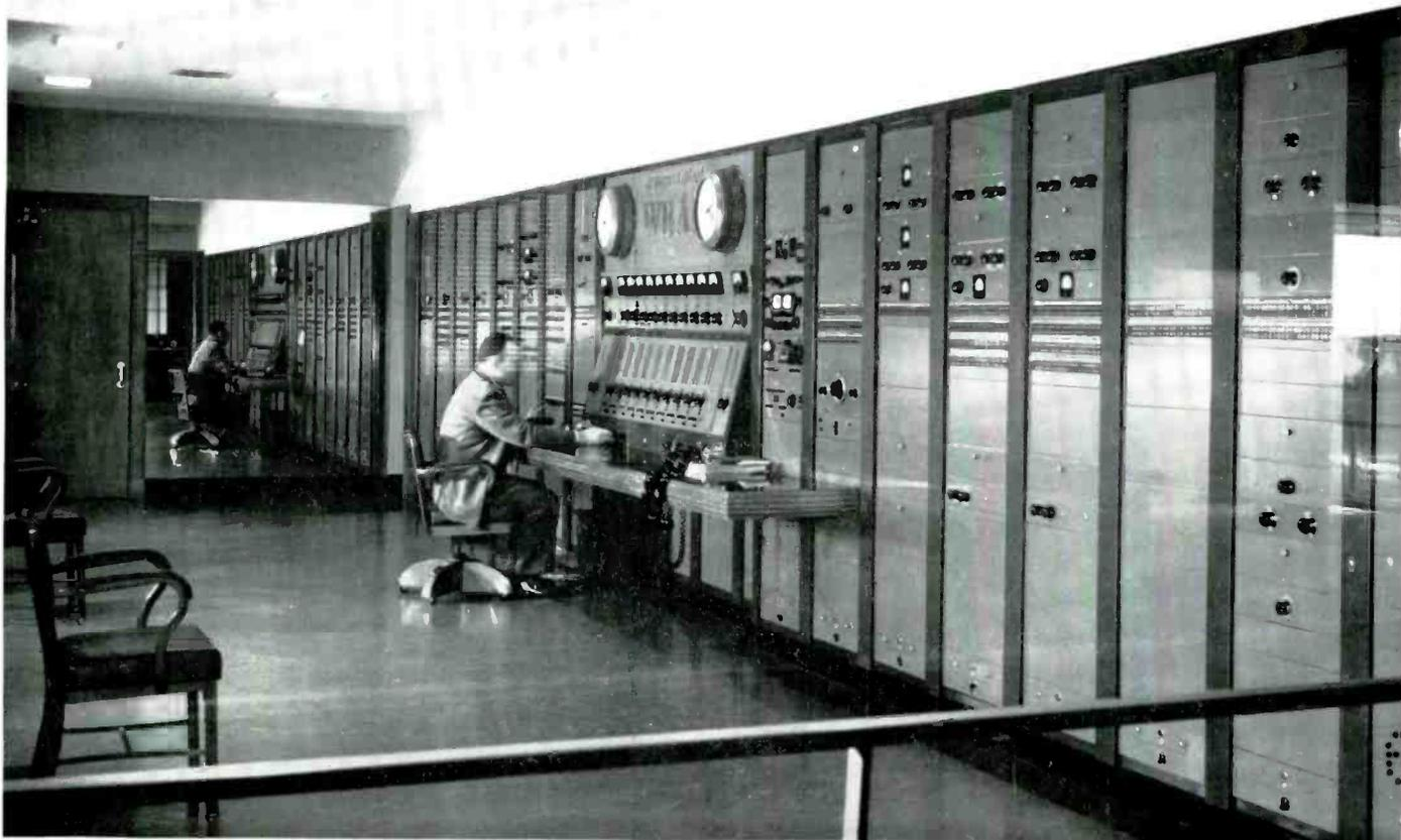
FIG. 33. View of WBAP's AM-FM Master Control Room as seen through the window from the main lobby. Twenty racks of equipment (with the main control position in the center) line one side of the room. The opposite side of the room (left in this view) is made up of three huge floor-length observation windows which divide the master control room from the corridor which runs across the front of the building (see floor plan, Fig. 6).
