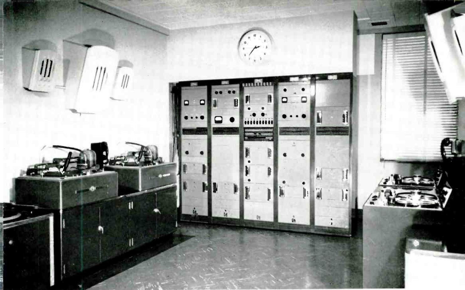
FIG. 31. WBAP's recording room is one of the finest station recording setups in existence. At left, in the view above, are the RCA 73-B Professional Disc Recorders. At right are two studio-type tape recorders. Racks in the center house line amplifiers, recording amplifiers, monitoring amplifiers, power supplies, switching facilities and the auxiliary equipment.
