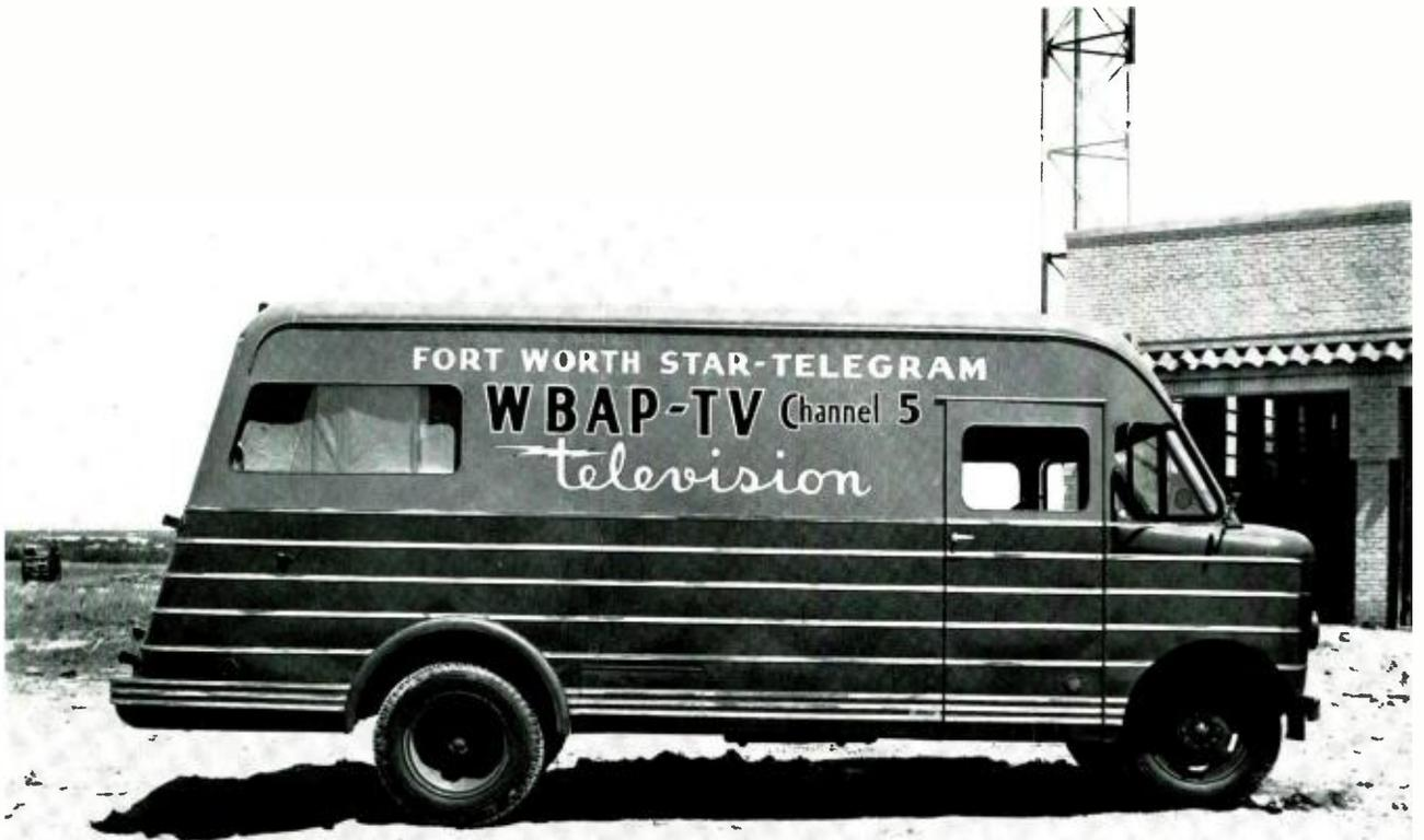
FIG. 21. WBAP-TV's field unit is an RCA TV-50A Mobile Unit with complete equipment, including RCA TK-30A Cameras and RCA TTR-1A Microwave Relay Equipment.
