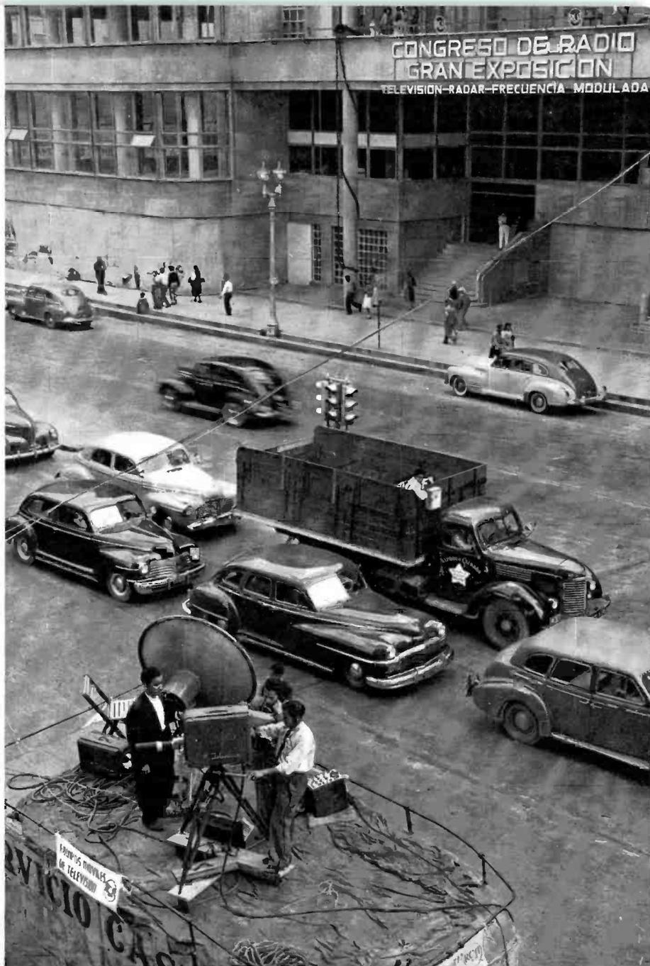
up the side of the stadium. The transmitter control and parabola were set up on a parapet near the rim with the parabola facing out through a "porthole" in the big concrete stadium. This location was direct line-of-sight from the hotel across Mexico City. First contact was made with the hotel roof by Morse code flashing light—until telephone communication was established—as both dishes were oriented for maximum signal from the three-degree beam.
