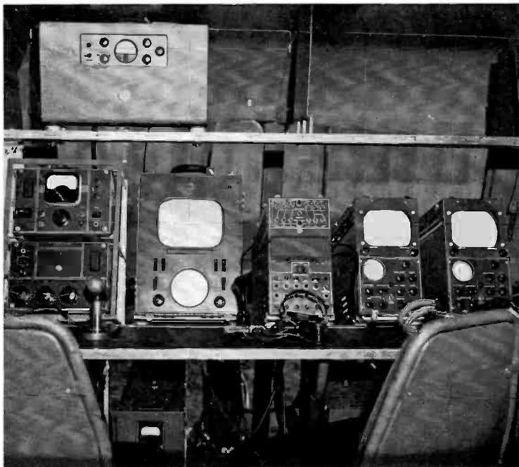
FIG. 2. (Left) The field equipment as it appears when mounted in the television truck illustrated on the opposite page. The units shown are the same as those identified in Figure 1 (above), with the addition of the two audio units (the well-known OP-6 and OP-7) at the left of the monitor and the microwave relay transmitter control on the shelf above.
