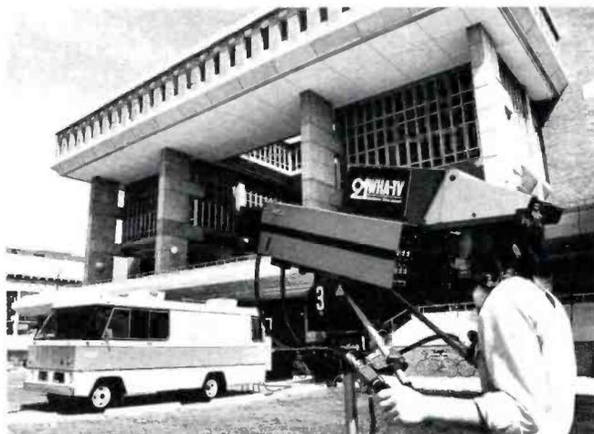
WHA-TV's mobile unit is a compact converted motor home. Widely used for instructional programs and documentary production, it is equipped with two TK-630 cameras and helical scan VTR's. Other van facilities include 8-input audio mixer; 8 x 4 video switcher with Chromakey capability, and portable microwave. The building in the photo is Vilas Hall.
