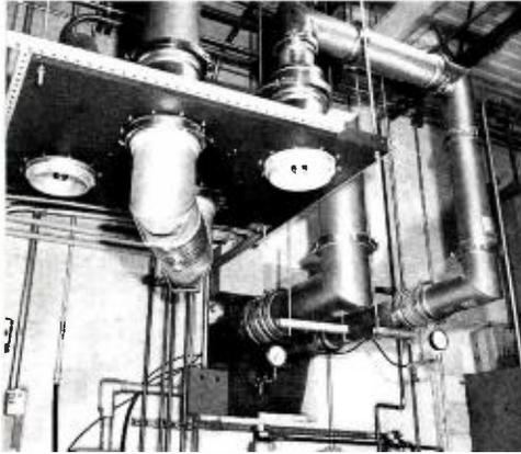
Manual coaxial patch panel for 9-inch transmission line to antenna.
