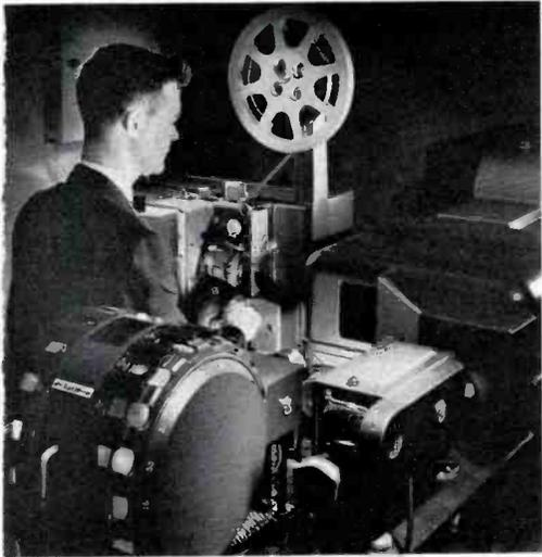
FIG. 7. Ken Foster threading 16mm TV film projector in Telecine room.
