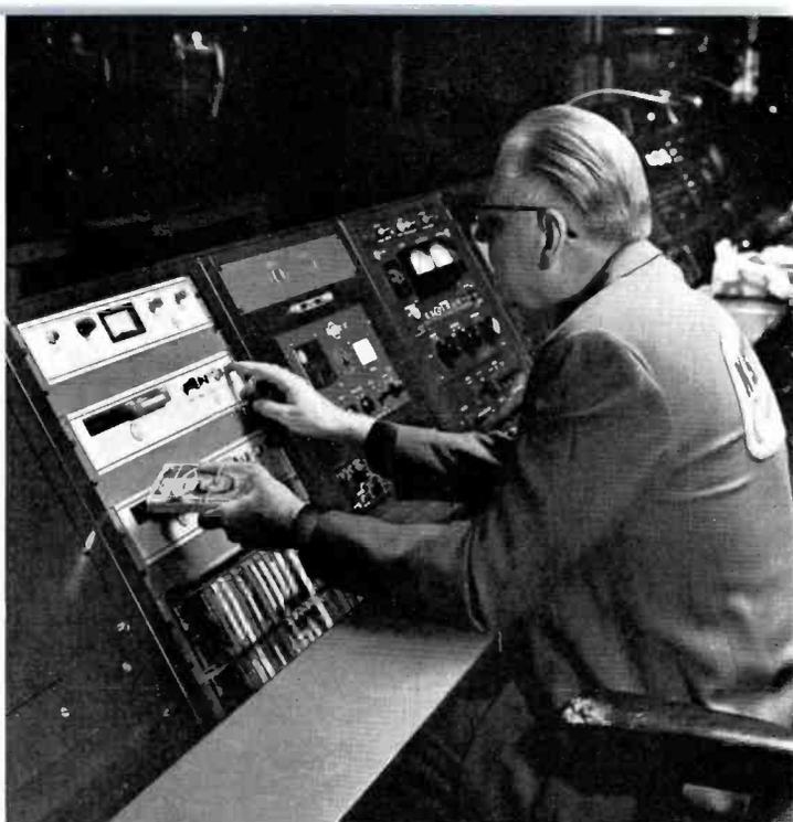
FIG. 26. RCA Cartridge Tape installations at master control. These units are tied into the automation system. Announcements are pre-recorded and started automatically for use with film and slide video. Ray Aula is loading a tape cartridge into the system.
