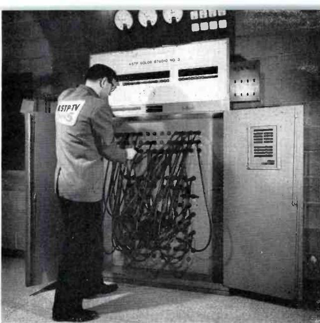
FIG. 14. (left) Three meters at top are load current indicators for the 3 phases on the 24 non-dim 50-amp circuits. Group of 12 meters and onboard panel are metering and control for 12 dimmer 50-amp circuits. All dim and non-dim circuits appear at top part of patch panel, while the 85 load circuits appear in lower part.
