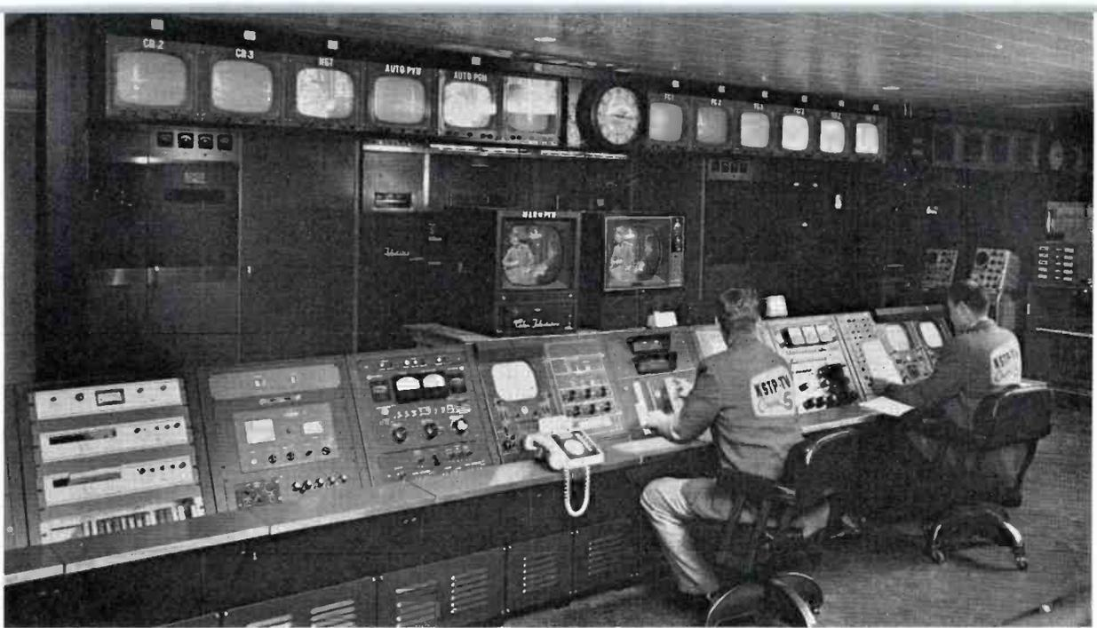
A great deal of editing and splicing is done. It's not unusual to run 20 splices in a half hour show. The Christmas color special, for example, included 50 splices. All of these are made with the regular RCA TV Tape splicer but with a KSTP design mounting bracket—for "sit-down" use.
