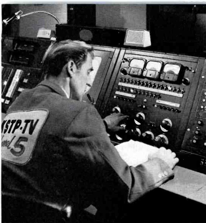
FIG. 25. View of the master control operating position showing master control audio. Bob Winters is at the controls. To his right are multiplexer and TV tape control panels. The audio control system was custom designed by RCA to meet KSTP requirements.
