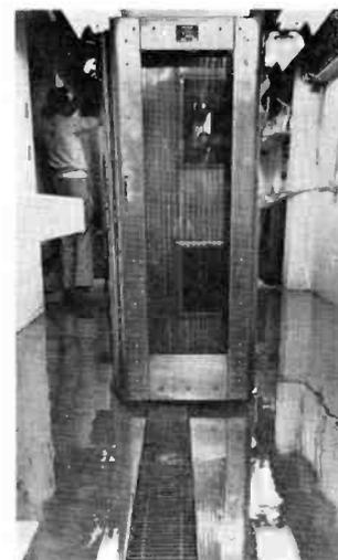
FIG. 60. Note floor drain system beneath film processor.
