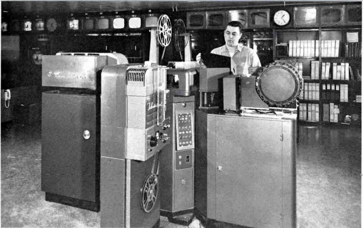
FIG. 40. Don Kline, projectionist, at Film Island No. 1 which includes two TP-6 16mm projectors and a TP-7 slide projector. Also TK-26 Color Film Camera, TP-15 Multiplexer, and TK-21 B & W Film Camera.
