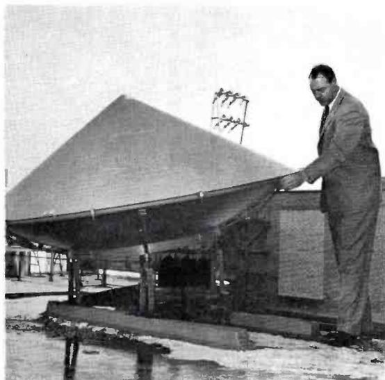
FIG. 46. Passive reflector is mounted at 250-foot level of KSTP tower.
