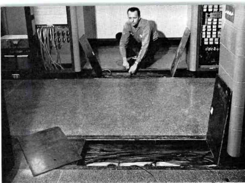
FIG. 29. Don Benedict pulling wire into trenching system. Trenches are under transmitter, consoles, and all racks. All run north and south and are 6 inches deep and 18 inches wide. Since area is designed with cellular metal flooring, cross access trenches are not necessary. Four-inch diameter holes (foreground) lead from trenches into cellular flooring and wires can be pulled down through these holes up into the selected trench.
