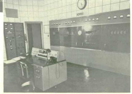
Here is the inside of the building showing the 5,000 watt transmitter installation.
