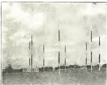
Painted yellow and black to reduce flying hazards these poles are used for the antenna installation at KDKA. The transmitter house shown in the preceding photograph may be seen in the background of this picture
