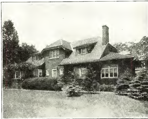
Fig. 1. Homes of this type lend themselves readily to the placement of radio outlets in each of the rooms with the receiver in a central location. The work may be done either while the house is in the course of construction, or else after the building has been completed
