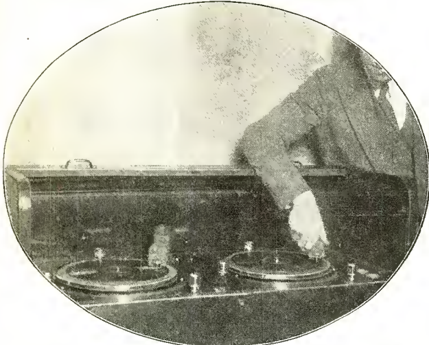
A system whereby radio broadcasts are transcribed on vulcanite or wax discs for simultaneous use by broadcasting stations is the accomplishment of John R. Kiel, 25 year old radio mechanic, who has perfected a machine which will make possible radio programs of a higher type, without the necessity of transmission by wire
