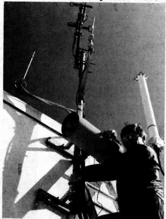
Ron, KB5BB Club secretary, installing remote weather camera at ATV repeater site.
