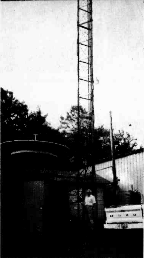
The W5KPZ ATV repeater tower in Tyler, Texas.
