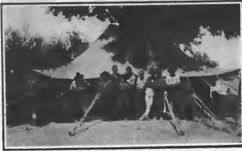
Field Wireless Station at Wadi Jemmami.
