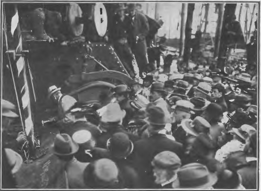
Laying the Keel of "Commonwealth Ship No. 3"
