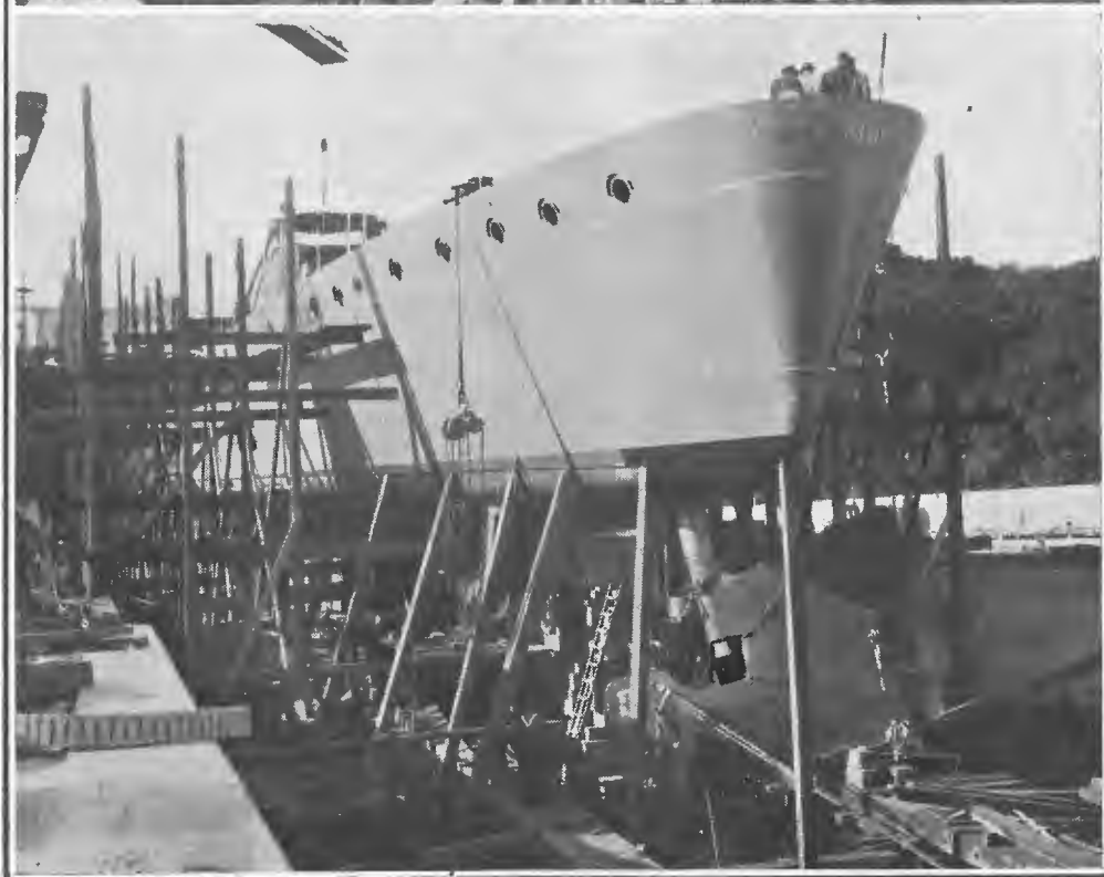
May 2, 1918.—The Stern Completely Plated (165th Day). July 4, 1918.—Fixing Rudder in Position (228th Day).
