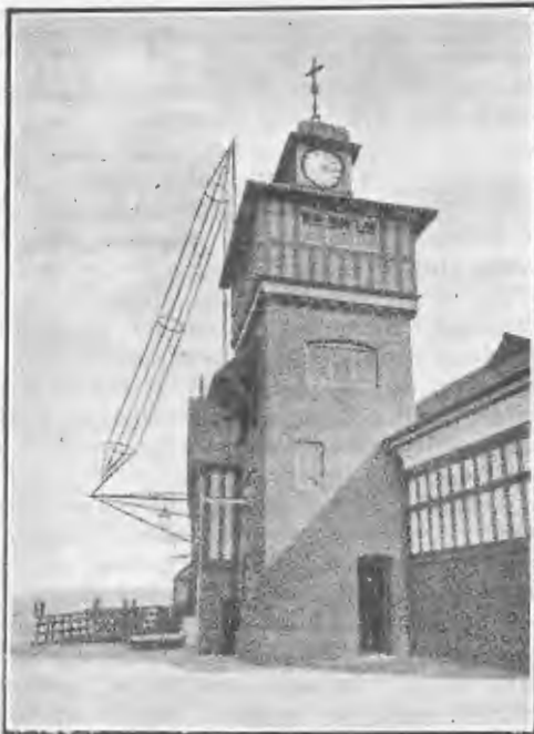
Automatic Wireless Fog-Signalling Apparatus Installed on Gourrock Pier, Glasgow. Note the Simple Aerial Arrangement.
