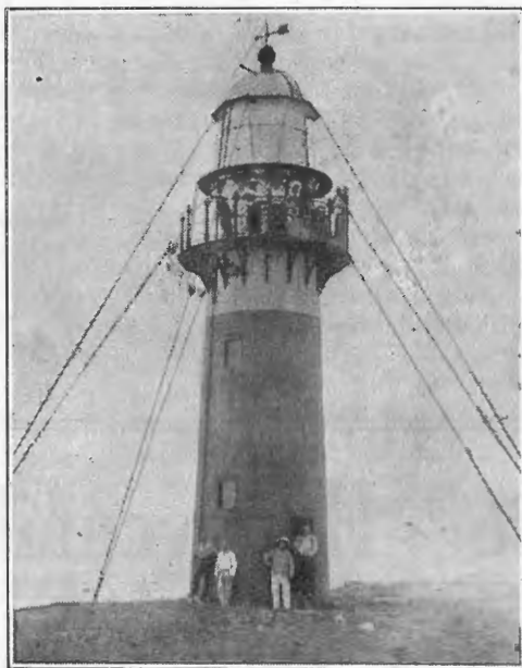
Jarman Island Lighthouse, off Cossack, W.A., is built of iron, and weighs many tons. Note the stays to prevent it being blown over by a "willy-willy."
