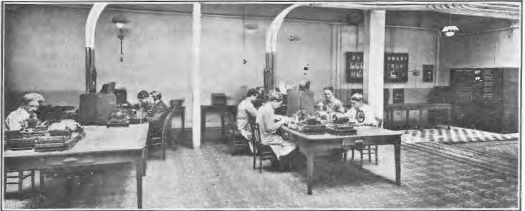
Operating room of Paris Radio Central. By means of long-distance control these operators work the actual station at Sainte Assise, twenty-five miles away.
