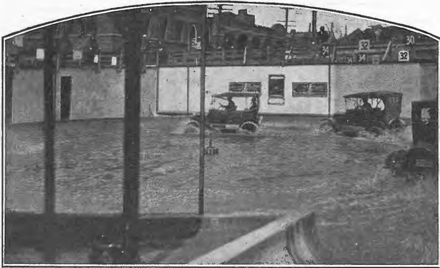
This huge concrete wash basin is the bathroom for many cars in one of the principal American cities. Payment of the equivalent of one shilling permits a drive round and round the basin to enable the undergear of the car to be well washed. An attendant first places a rubber sheet across the radiator to protect the "maggie" from the splashing.
