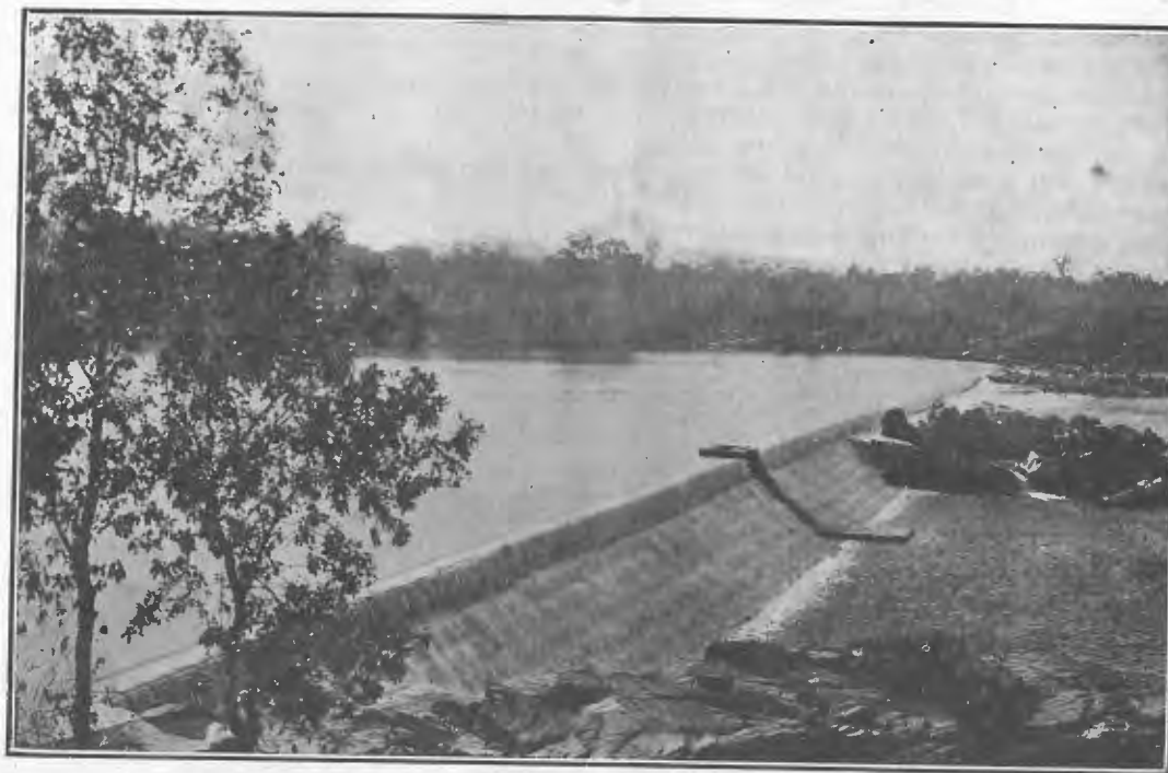
Near view of the weir, Burdekin River, Northern Queensland.
