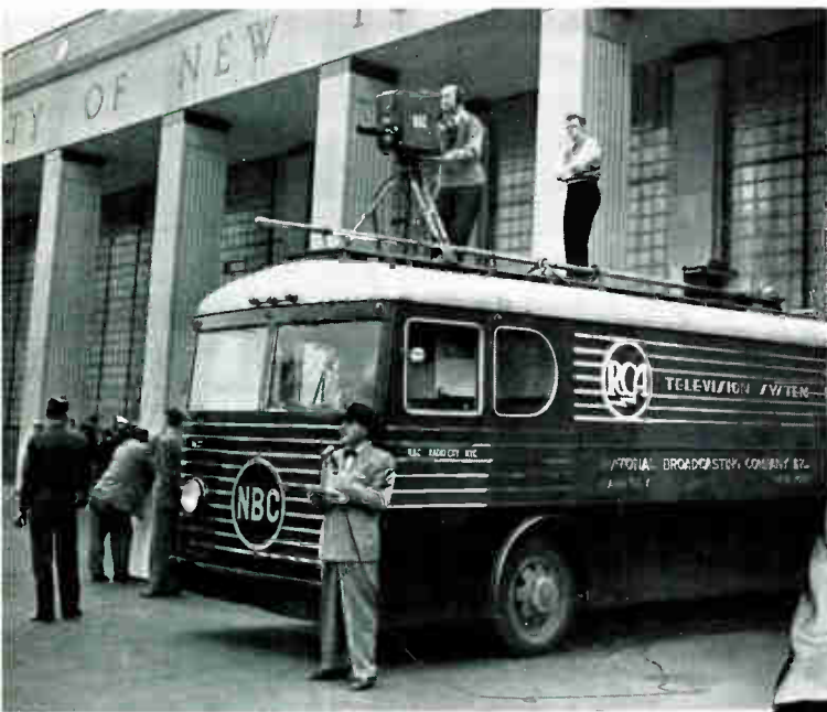
News events are televised from a special truck carrying crew, cameras and microwave relay equipment.
