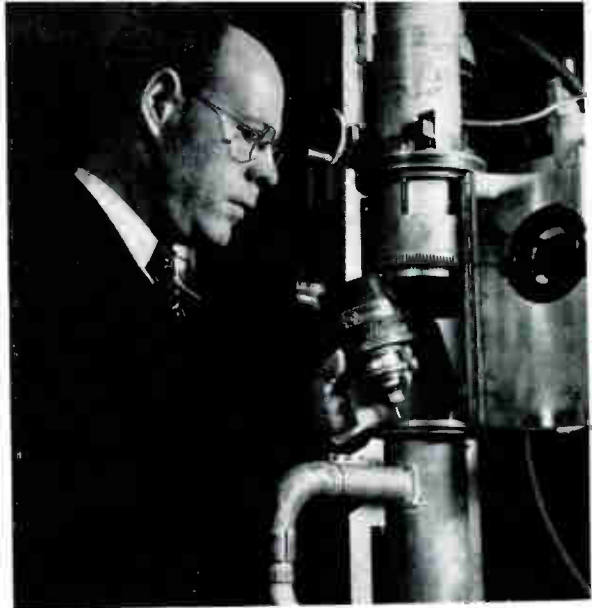
Inserting a high-power, high-frequency television transmitting tube in its housing.
