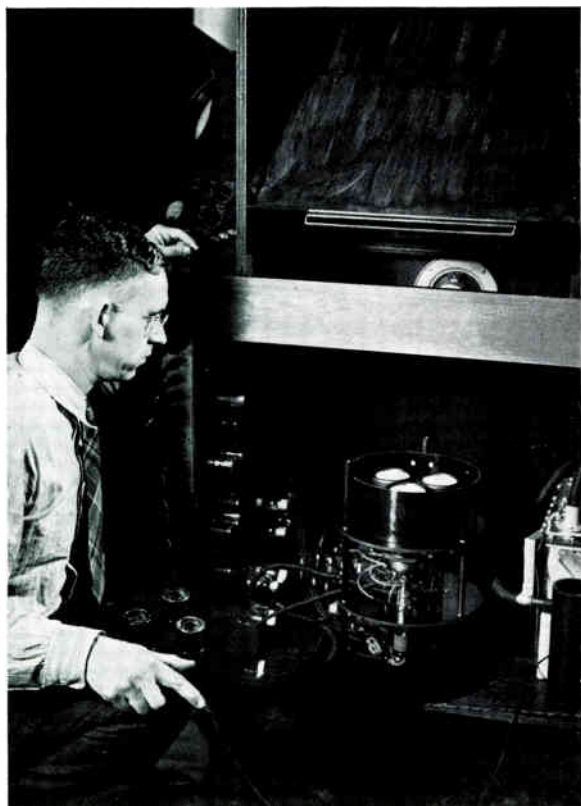
Trinoscope projector which makes possible reproduction of television programs in natural color by RCA's simultaneous all-electronic color system.
