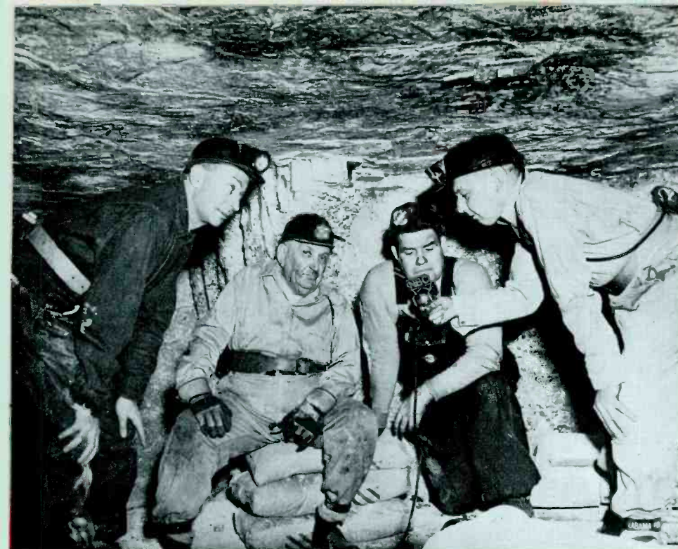
Conducting radio interview in an Alabama coal mine.
