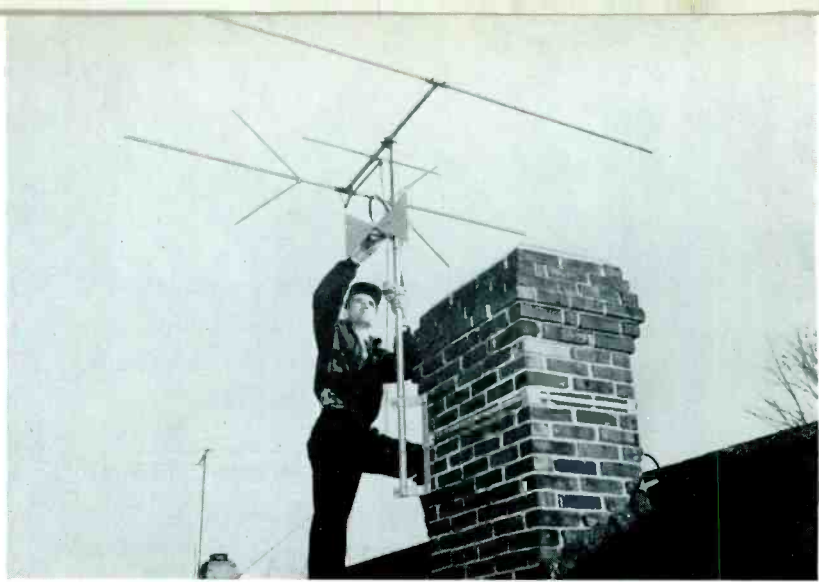
Service Company technician installs UHF-TV antenna.
