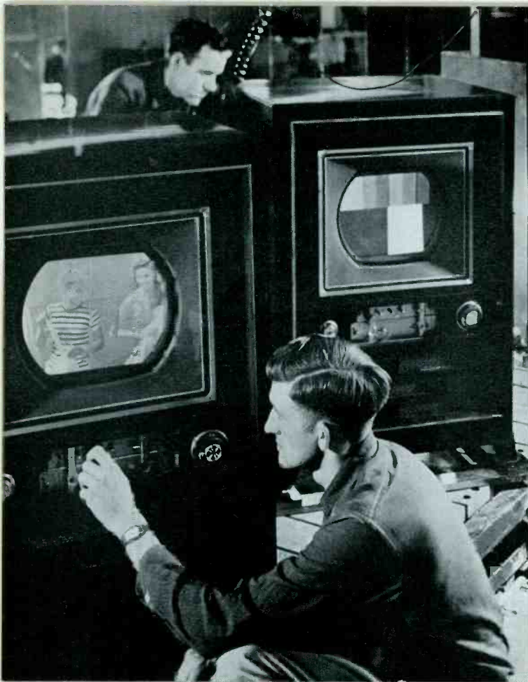
Color slides are used to test color set performance.
