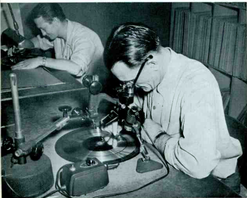
Technician checks master record with a microscope.
